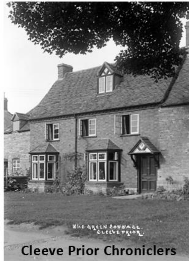
The Green Cottage, Cleeve Prior
