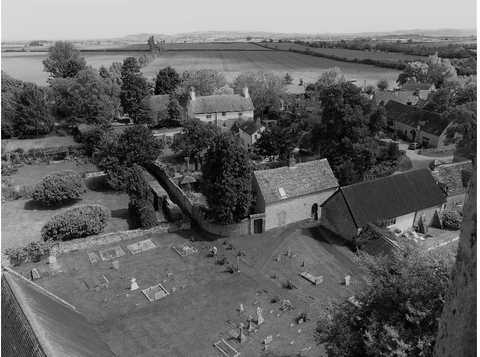
View from the Church Tower
