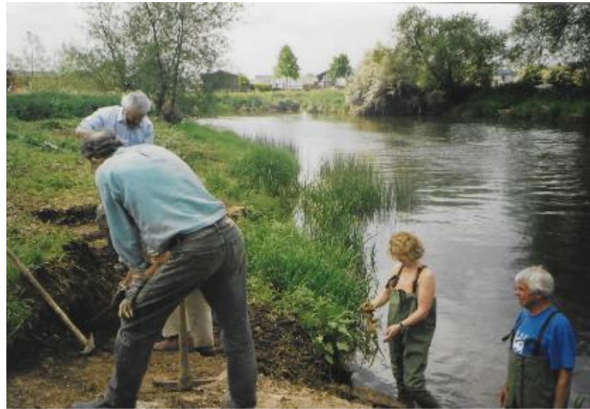
An area of the old weir face was exposed
