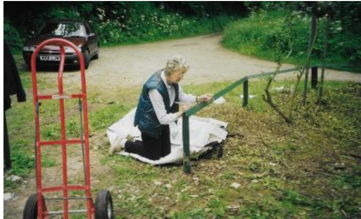
Fencing was repaired and the facilities improved
